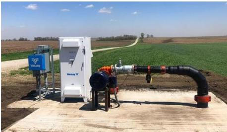
The other unit, an *EZY Switch* model **SMS-2**, is located at the Pumping Station. The SMS-2 controls the well pump via an integral relay contact output.
